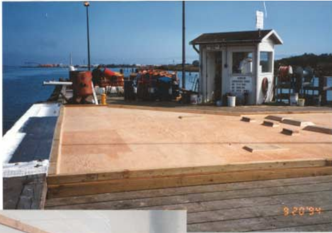
View of petroleum barge dock secondary containment area under construction using plywood sheeting and wood beams as base materials.
