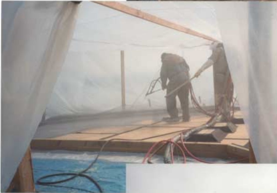
View of petroleum barge dock secondary containment area under construction using plywood sheeting and wood beams as base materials.
